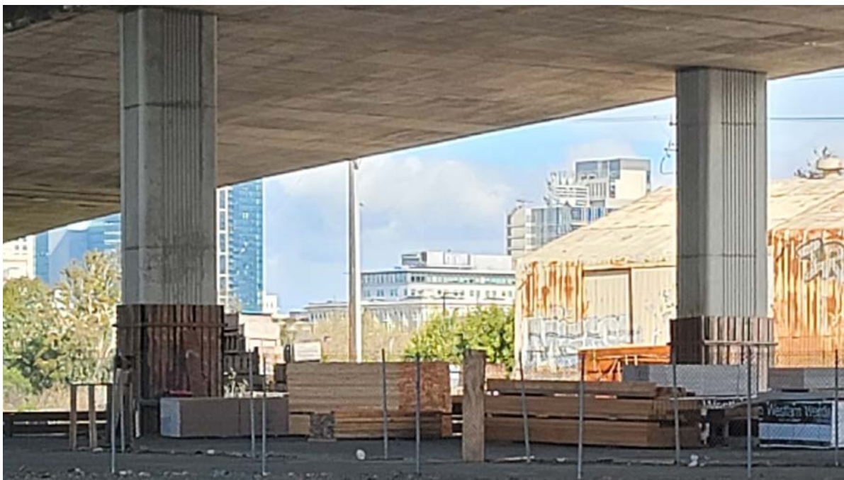
Photo 5. Oakland airspace underneath I-880 containing wood materials on March 13, 2025
